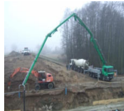
Technological suitability eg for backfilling with a concrete pump
